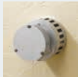
Balanced Flue (No chimney required)
