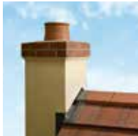
Brick/Stone Chimney (Class 1)
