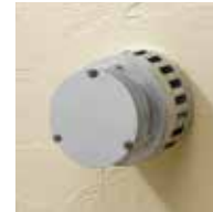
Balanced Flue (No chimney required)
