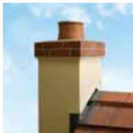
Brick or Stone Chimney (Class 1)
